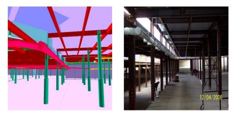
Figure 6 Visualizing the building before it's built - 5 month in advance
